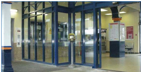
Platform/entrance improvements at Eastleigh have recently been completed to allow 24 hr access to the overbridge.
